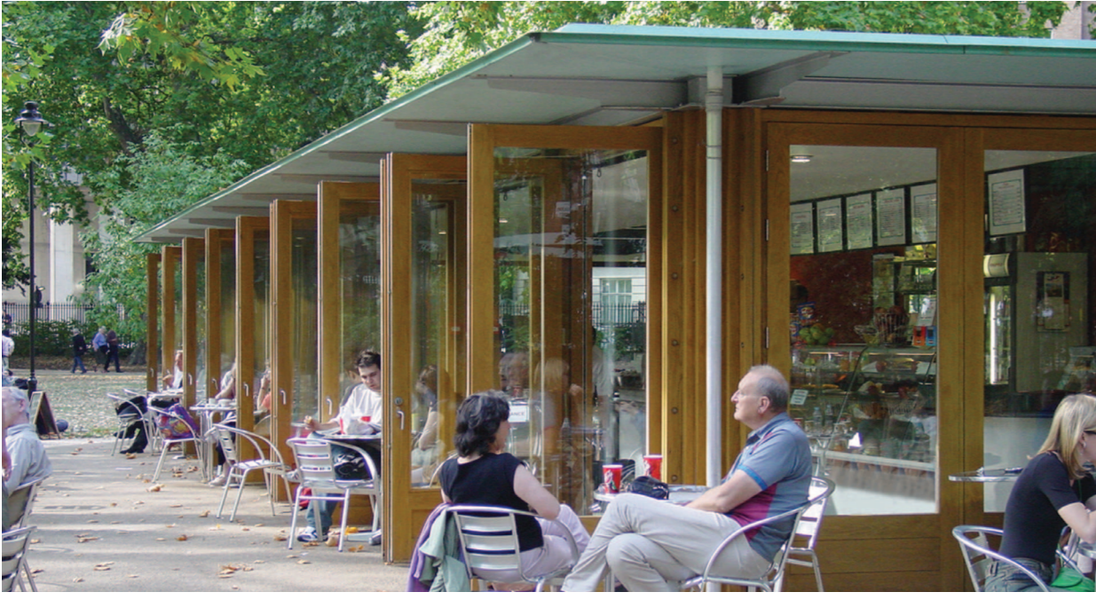
Low structures with overhangs
