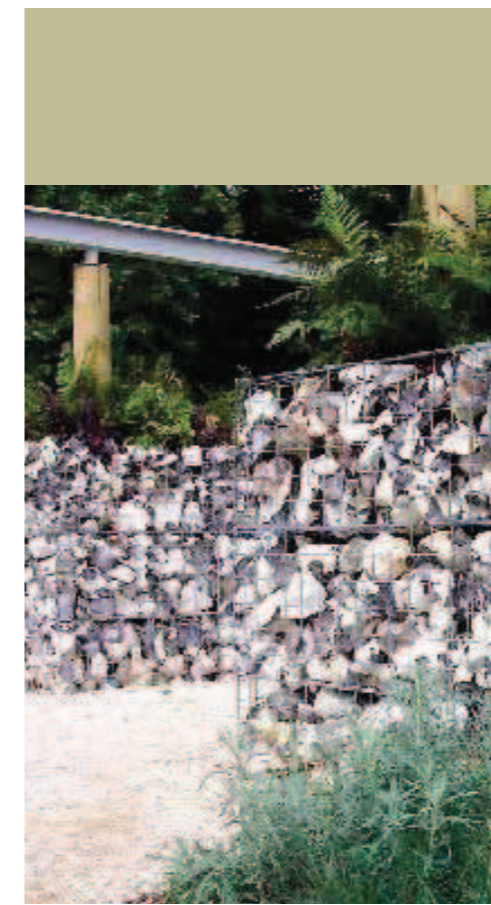
Flint gabion walls
