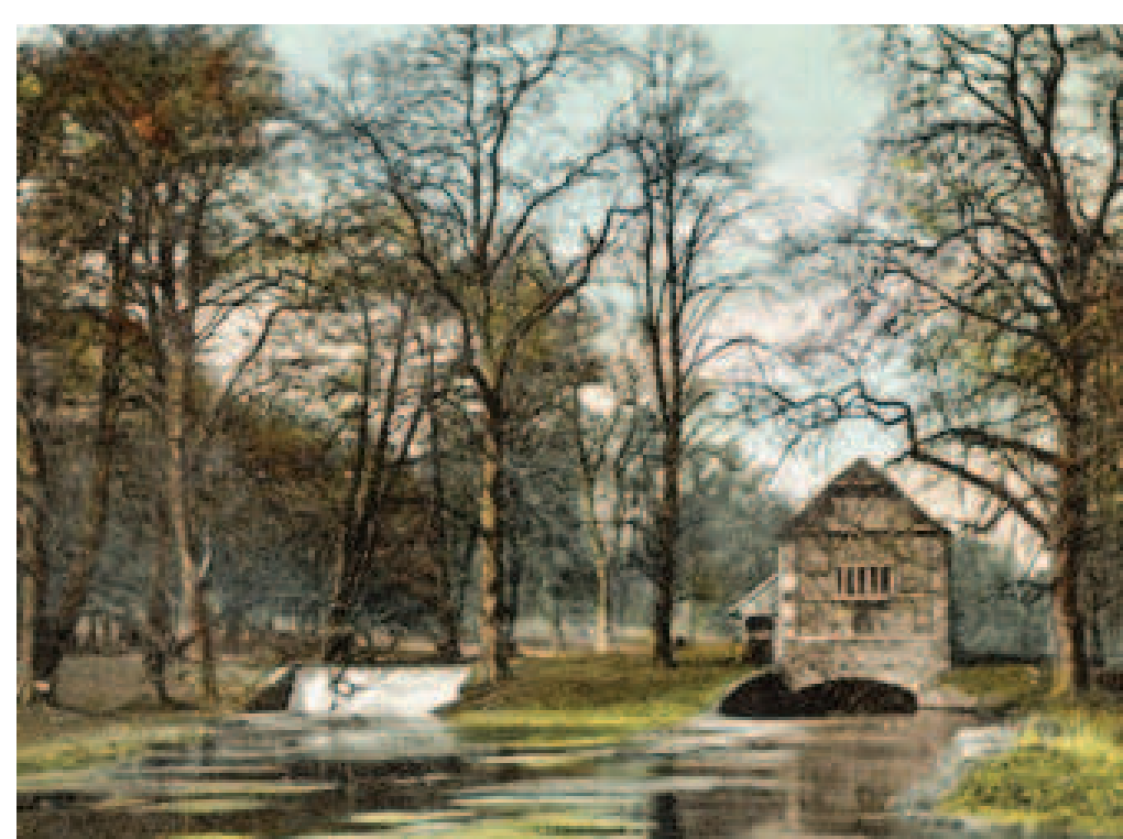
Restoration of open parkland character
